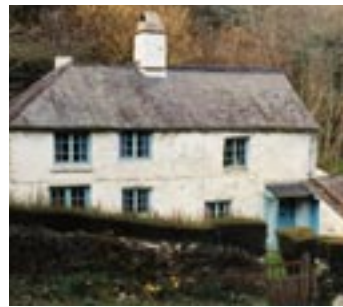
54 - Foxhole Cottage, Foxhole
