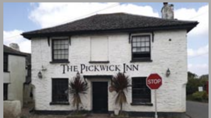
EXAMPLES OF LISTED BUILDINGS
